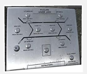
The crew member at the control console closes the gates by pressing and holding the 'Close Gate' button. Once the gates are closed, the lock must be emptied by pressing and holding the 'Let Water Out' button. To keep the boat steady as the lock empties, the bow and stern lines need to be kept taut during the whole manoeuvre.
